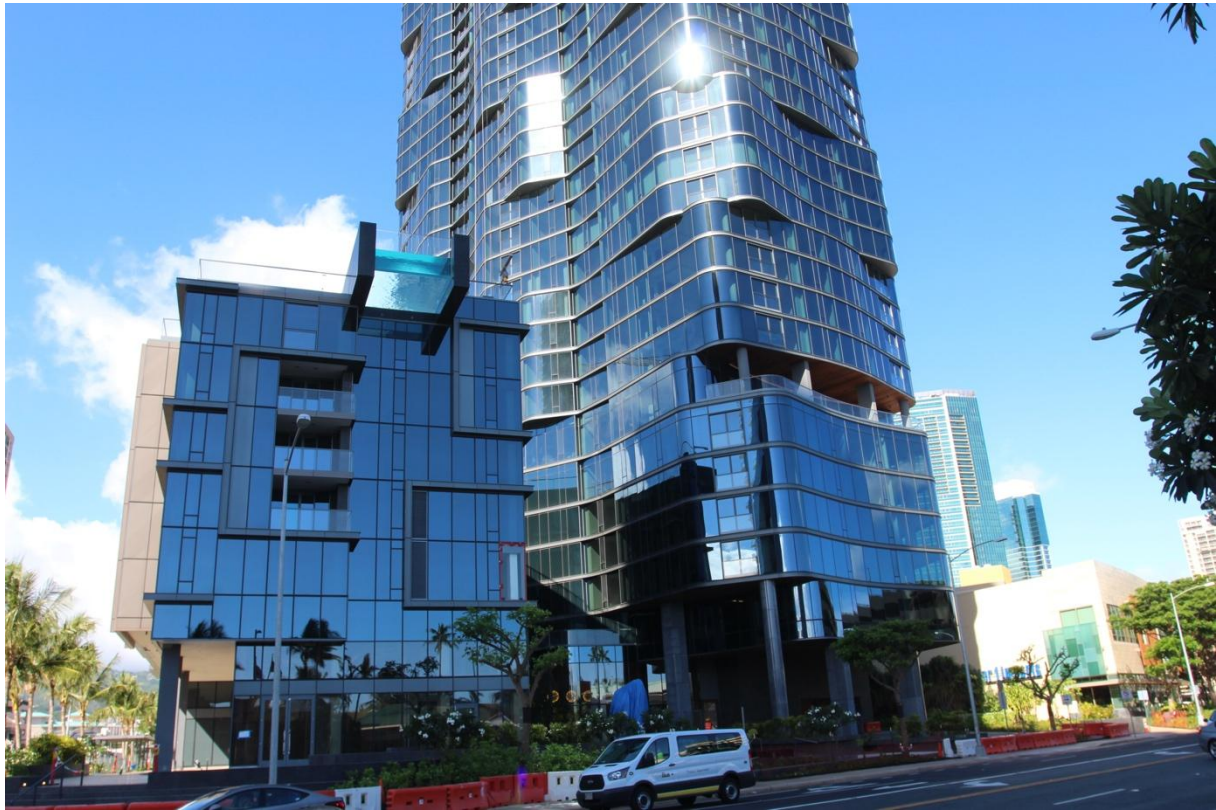
Figure 3 : Ward Village, Anaha © Holzinger, 2017
